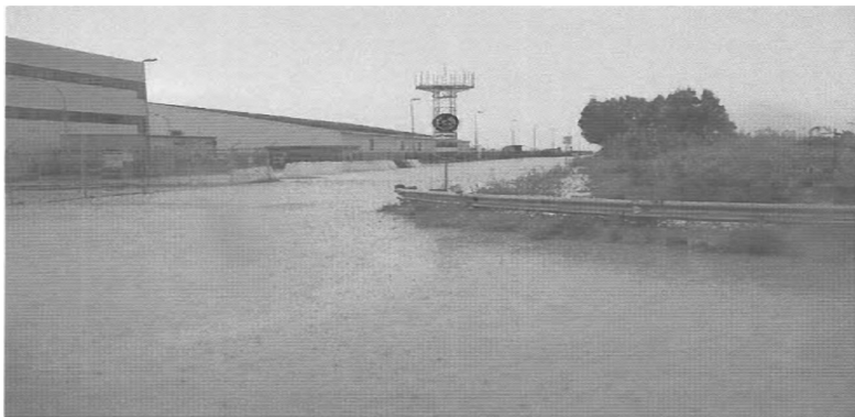
Sigonella Base after 13 December 2005 flooding
