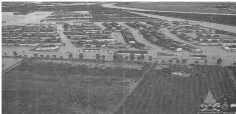
Marinai Housing after flooding of 13 December 2005 View from West
