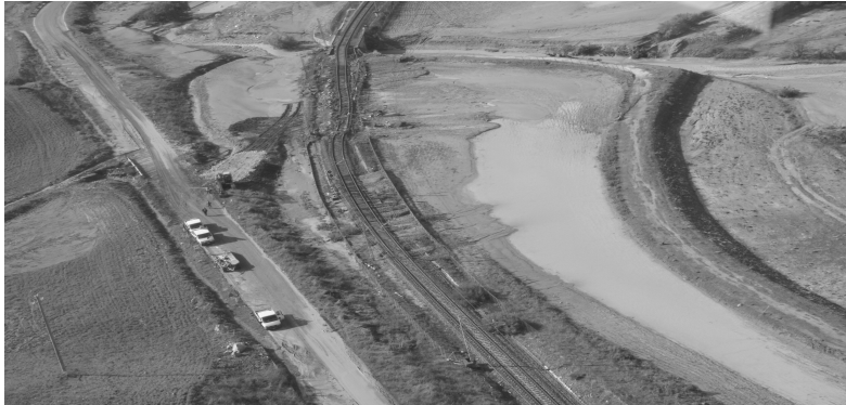
Simeto Basin – Damages to infrastructures from 13 December 2005 flooding
