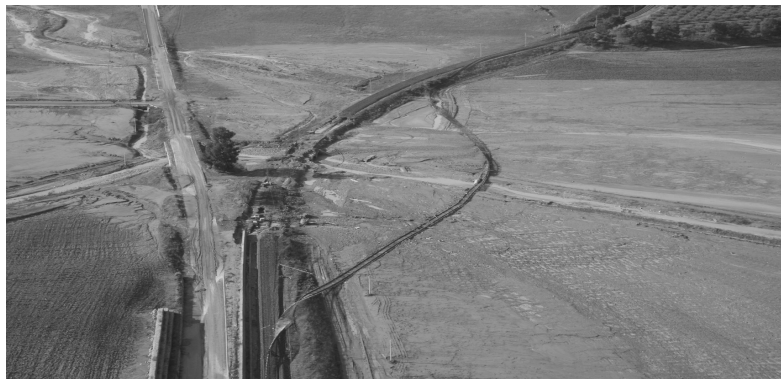
Simeto Basin – Railroad disrupted by 13 December 2005 flooding
