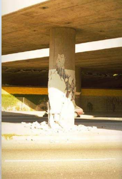
INTERSTATE-10/LA CIENEGA- VENICE BLVD. Northridge, California Earthquake, Jan. 17, 1994 M=6.69
