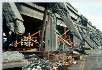
CYPRESS VIADUCT, INTERSTATE 880 Loma Prieta, California earthquake, 17 Ottobre 1989 Mag. 7.04
