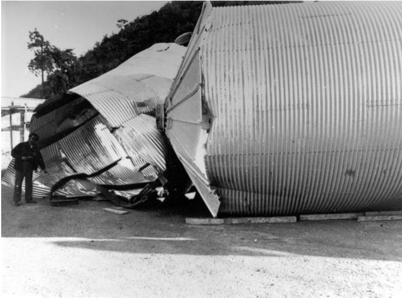
Guatemala Earthquake 1976. Collapse of a corrugated steel grain silo in Villalobos
