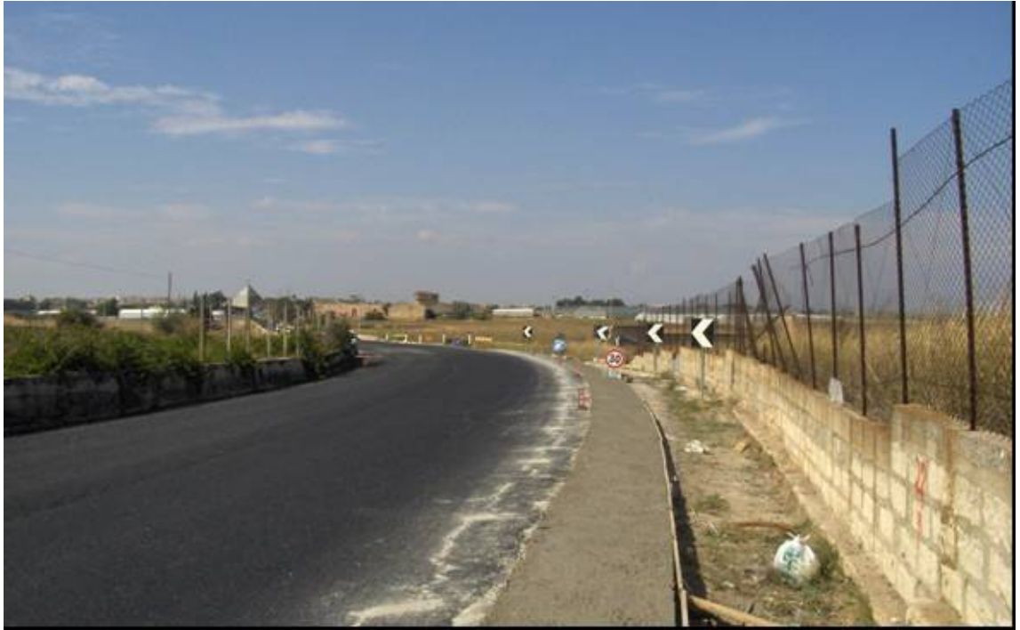
Figure 89 Creation of new shoulders/kerbs
