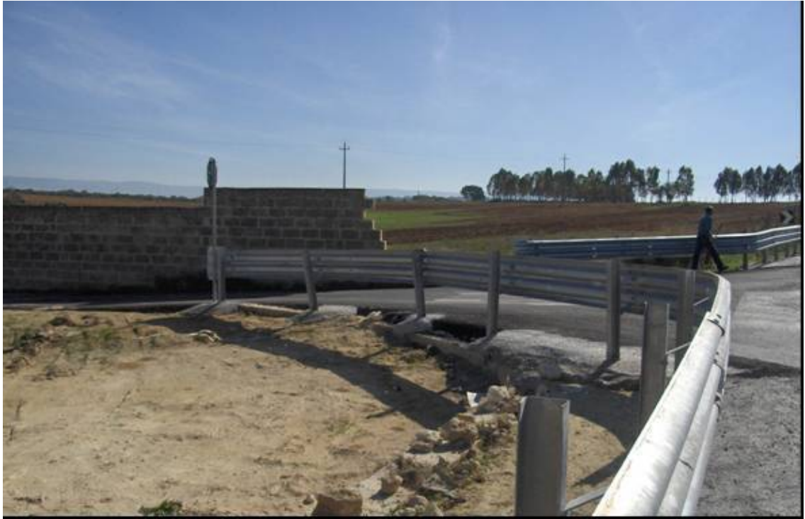
Figure 91 Repair and substitution with H2 type approved protection barriers
