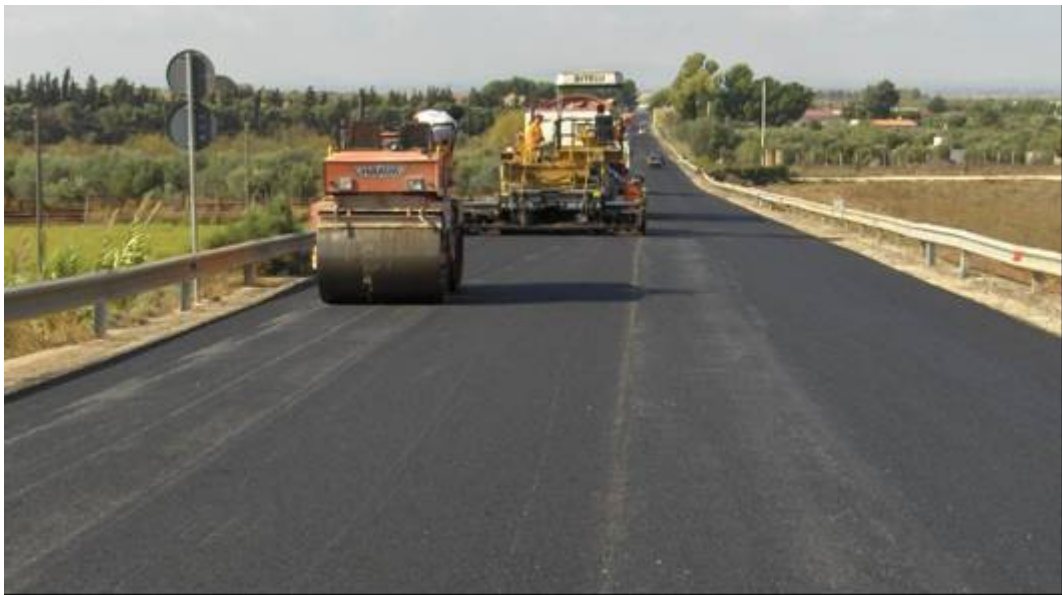
Figure 88 Resurfacing interventions
