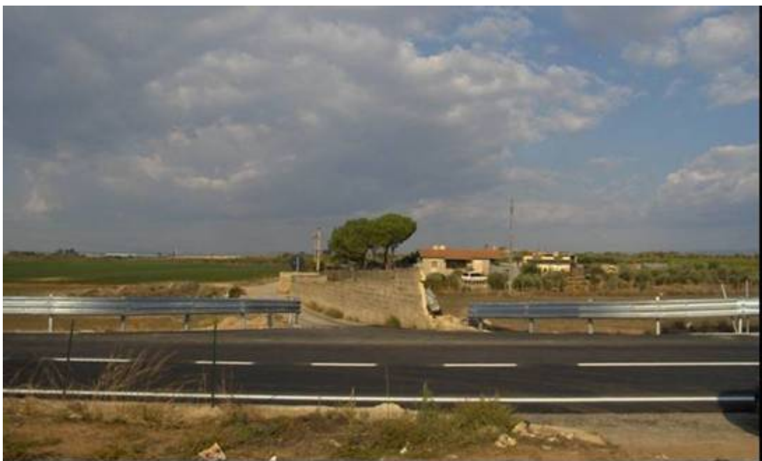
Figure 92 Installation of new barriers after building concrete kerb.
