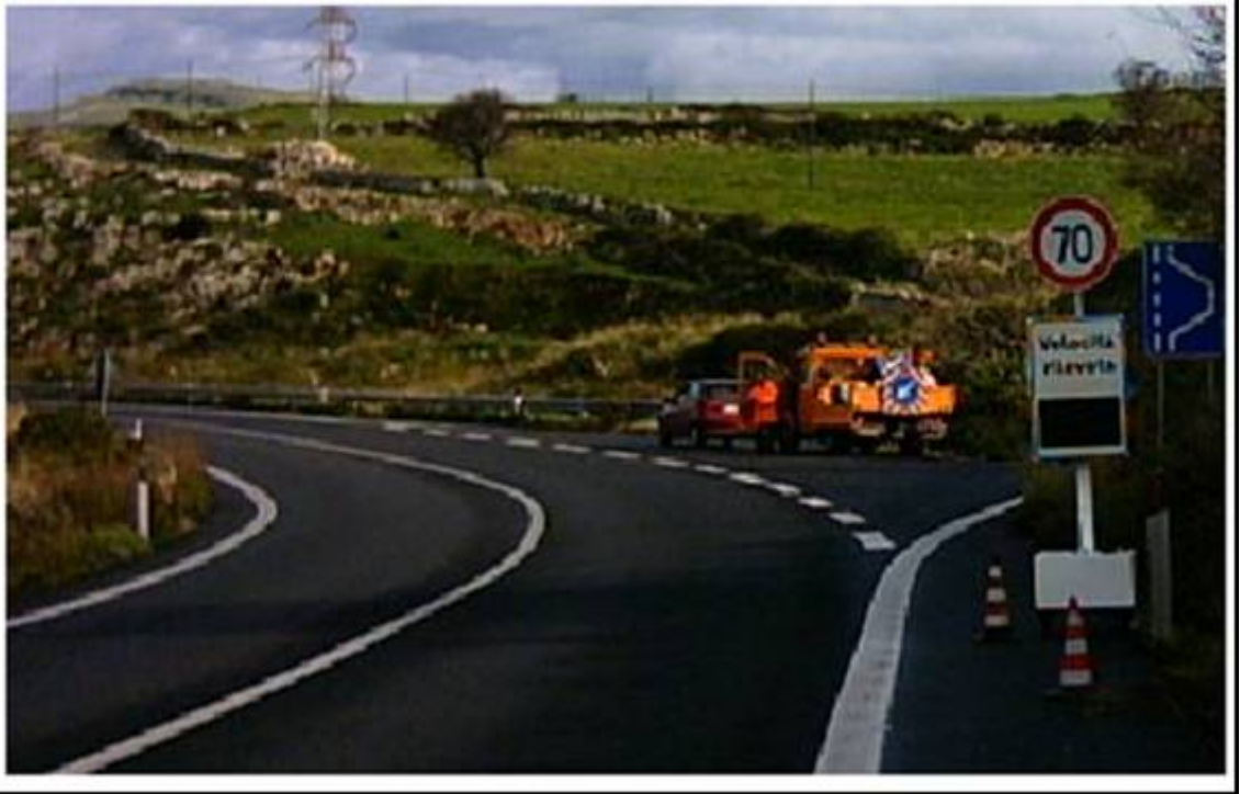
Figure 56 Positioning of the DFS with combined speed limit signal.
