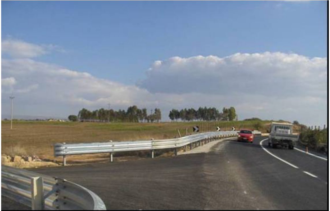
Figure 96 New shape of the barrier at the intersection
